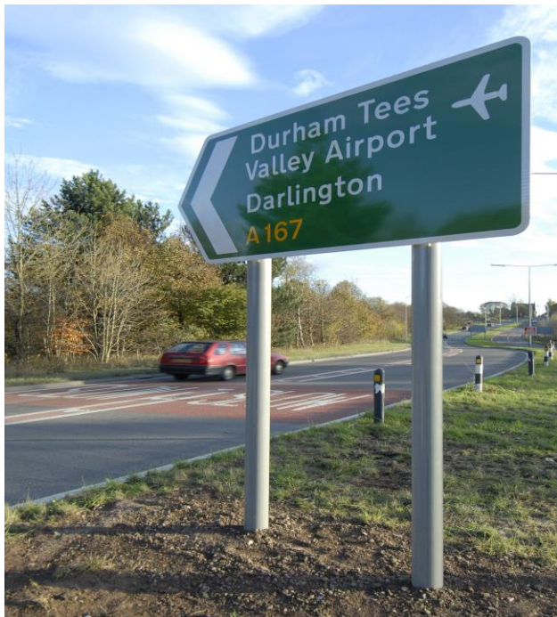
Typical installation of an FSP post
