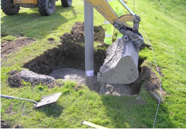
Direct burial installation as for steel posts.
