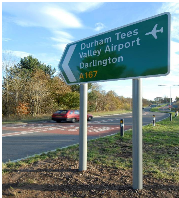
Typical installation of an FSP post
